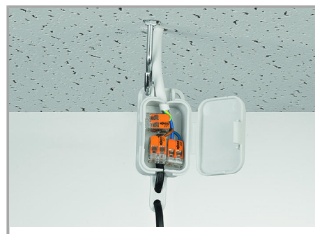
Pendant light connection in suspended ceilings
